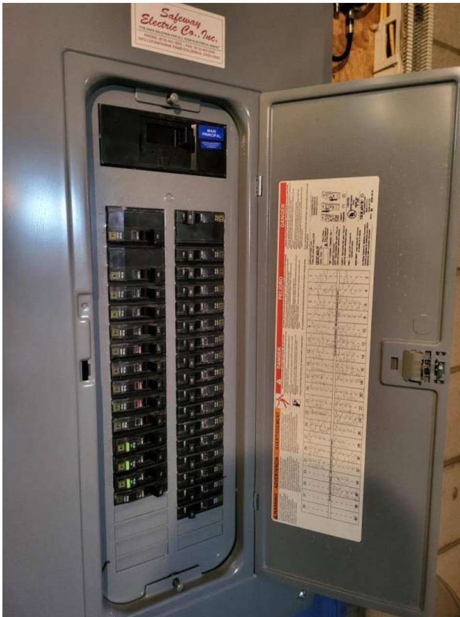
Single and/or Double-Pole Circuit Breakers.
